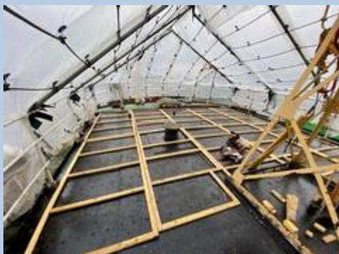
the bridge deck and is a major improvement. Wooden frames have been fabricated and these will be completed once lockdown is over. The frames will be fitted proud of the metal deck and will be used to support plywood sheets
